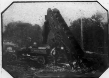
Grading Streets for Paving.
